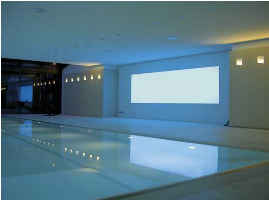
Swimming Pool Mondian: farbige Beleuchtung hinter Spannfolie. Swimming Pool Mondian: coloured lighting behind a foil.
